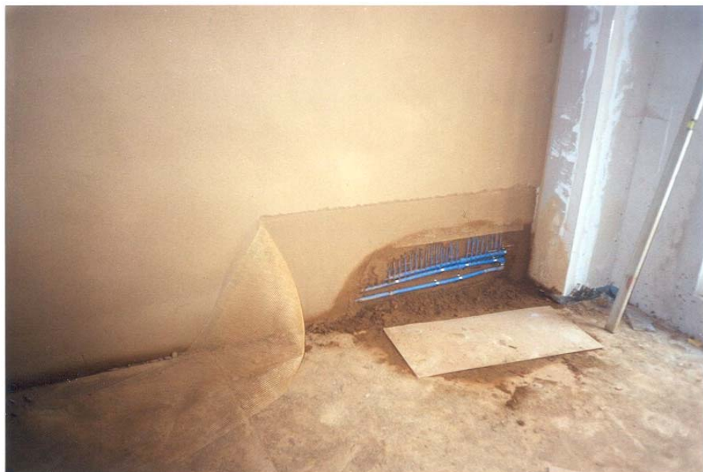
Picture 2: Earthen plaster on a wall-heating-system
