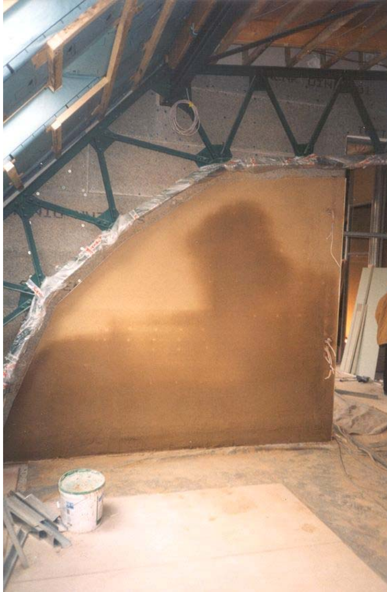
Picture 3: Earthen plaster for a favourable room climate
