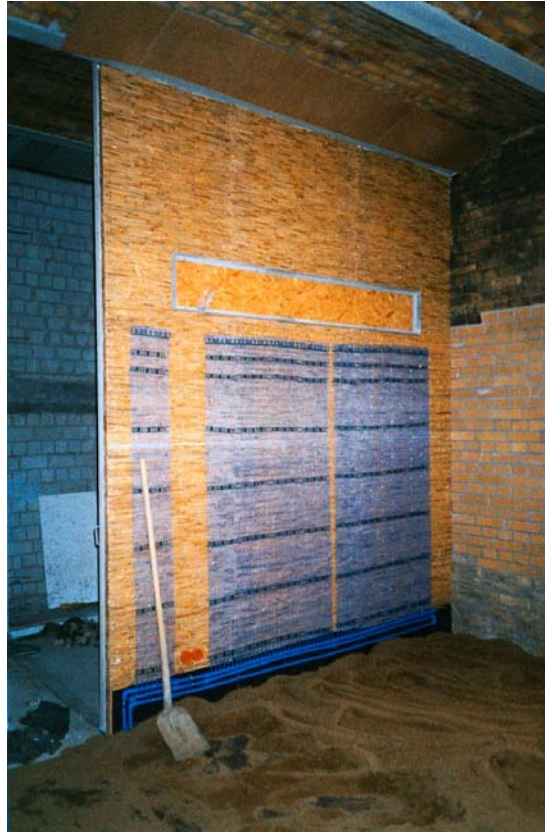
Picture 1: Preparation of a wall-heating-system
