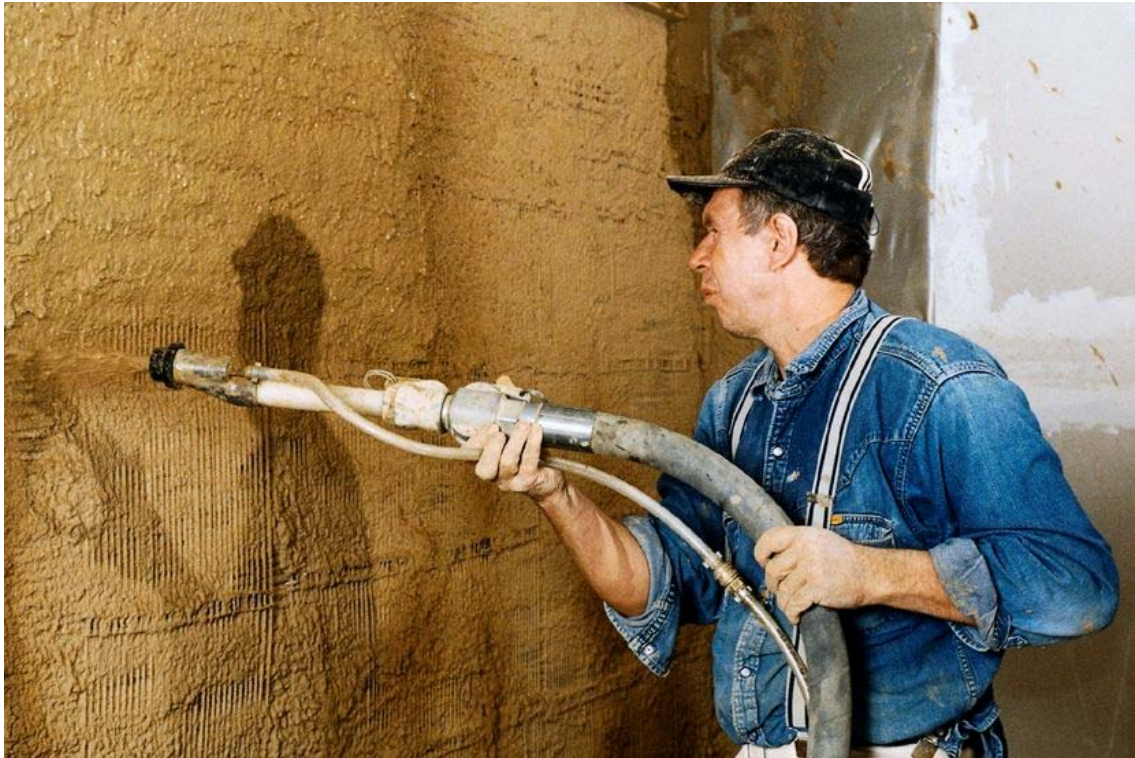
Picture 4: A vocational training in earthen plasters
